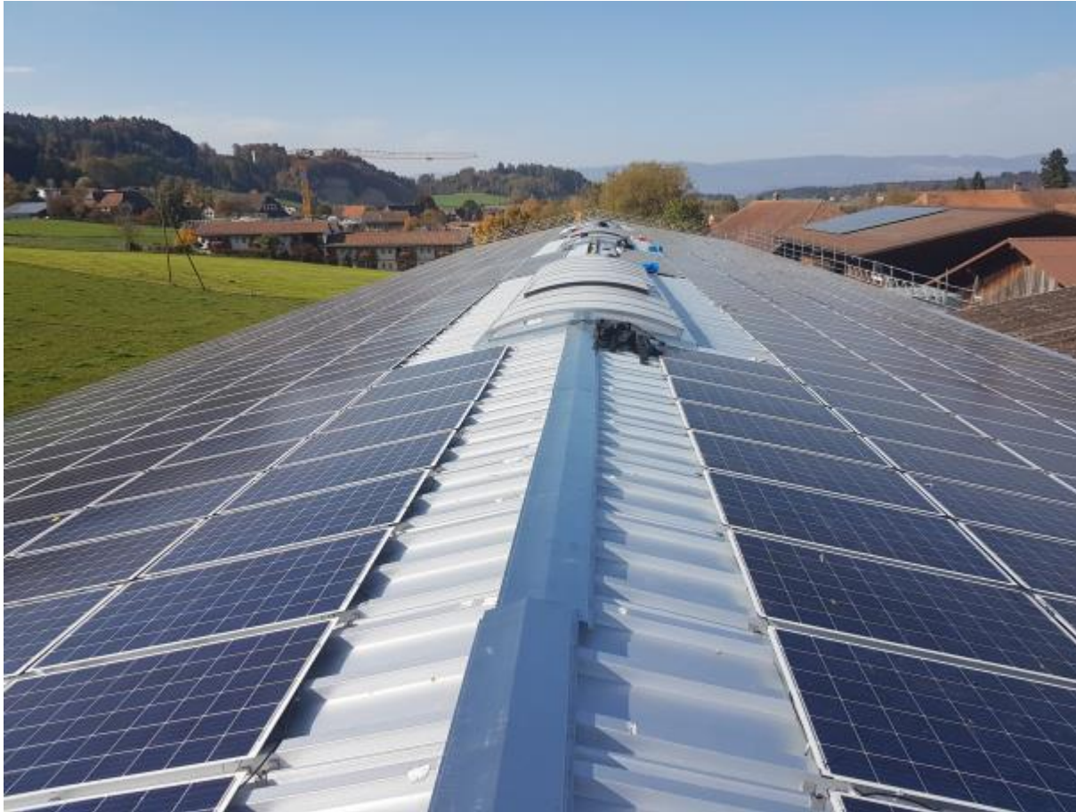
2000 sqm, 280 kWp, Bern - Production Hall – During installation
