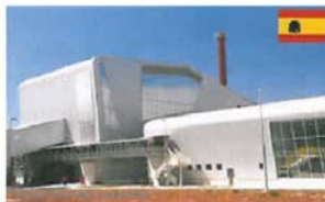
Sanguesa Power Plant
