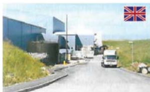
Elean Power Plant
