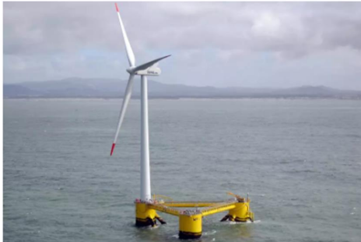
A floating wind turbine is pictured off the coast of Agucadoura, near Porto, in Portugal (AFP/Getty Images)
